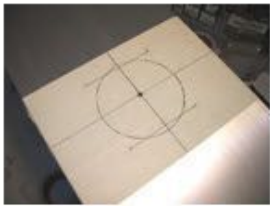
Use masking tape & ruler to measure location for 120mm cooling fan
